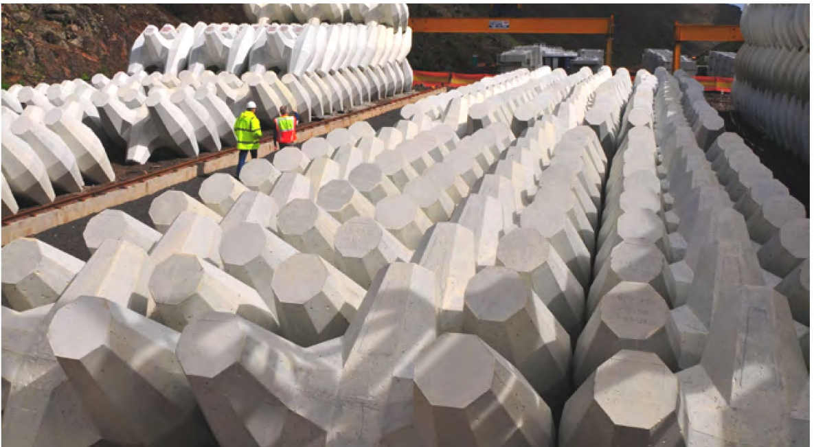
Over 700 units of precast Core-loc armour units (7 tonnes per unit) and hollow blocks (27 tonnes per unit before being filled with stone) were placed by crawler cranes via GPS around the wharf from the surface bed to just above sea level.
